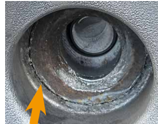
Photo 8. Too much impacting with an air tool can also crack the adjacent area around the nut
