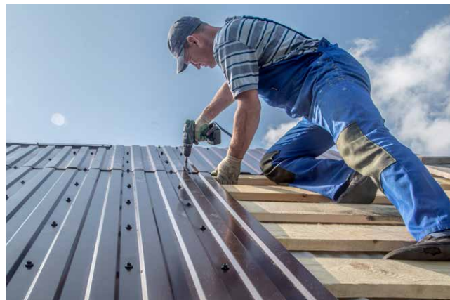
Figure 3: Installation of Exposed Fastener Metal Roof System
