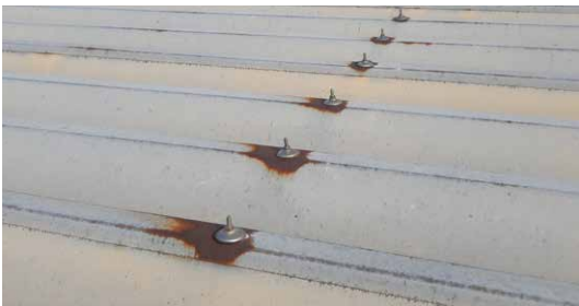
Figure 6: Example of Corrosion to the Head of the Fastener and the Metal Roofing Panel
